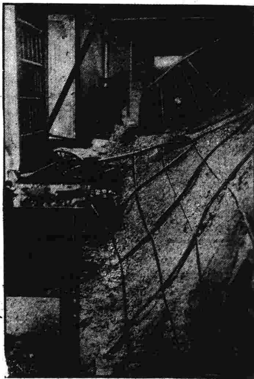
An office in Cleveland Clinic hospital which was wrecked by an explosion and fire that took toll of more than 100 lives, is shown above. Spectators said they saw the roof of the building lifted by the force of the blast.
